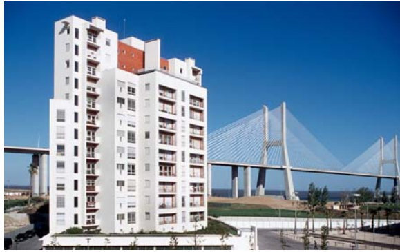
Figure 5d: Torre Verde (Green Tower), an energy efficient twelve-storey residential concrete building (7,200 m 2 ), constructed in Lisbon, Portugal. Monitoring has shown that it emits around 24 tonnes less CO 2 per year than a conventional building of the same size. The solar thermal system supplies 70% of the heat required by the domestic hot water consumption of the building. (Courtesy of Tirone Nunes, SA, Portugal)
